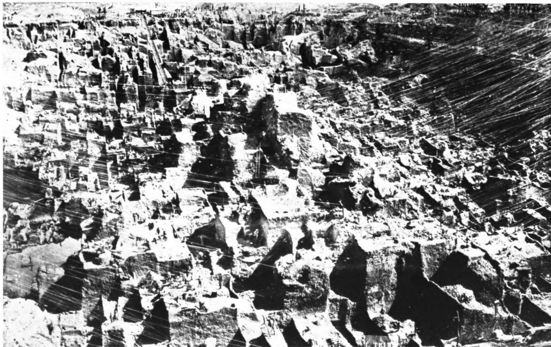
54 The Kimberley mine in 1877; the roadways between the claims have vanished and the scene is one of apparent confusion, with hundreds of claims being worked at different levels and a vast cobweb of haulage ropes
